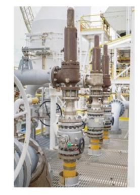
*Figure 4.2: PRVs are critical for* safety, but they can create maintenance headaches. They also tend to be at the high end of piping and vessels, so access is often difficult.
