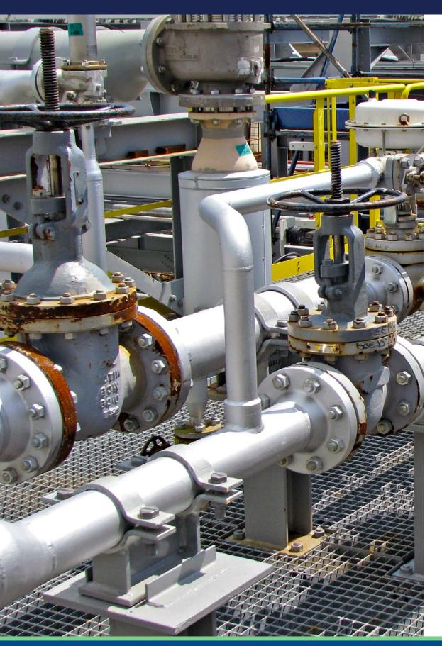
One source that feeds a flare, and may also be responsible for atmospheric releases, are pressure relief valves (PRVs, Figure 4.2). If the pressure of piping, a vessel, or reactor exceeds safe limits, PRVs open and allow pressure to reduce to an acceptable level. The PRV will then reseal when tolerable pressure levels are restored.
