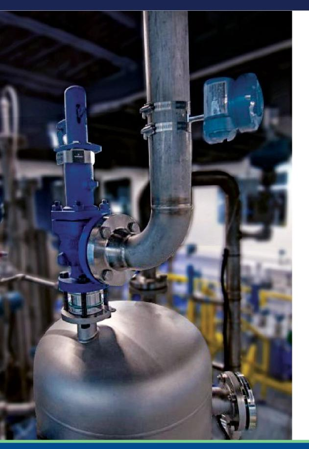
The challenge is identifying which valves are not working correctly. If operators want to know what is happening with a particular PRV, they typically rely on local inspection, or they monitor normal process pressure measurements for indication of operation near the PRV's setpoint.
