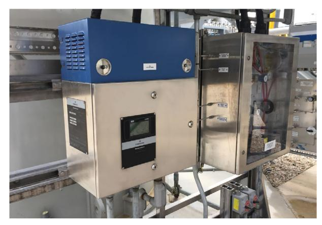
Figure 1.7: A hybrid QCL/TDL analyzer, such as Emerson's Rosemount CT5100 Continuous Gas Analyzer, can measure up to 10 gas components simultaneously in real time, from partsper-million (ppm) to percent concentrations. It is ideal for hot/wet CEMS applications and features a purged and pressurized enclosure for hazardous areas.
